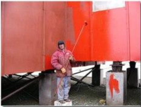
Alex, UA1PAW painting the building walls at Bellinghausen Base.
